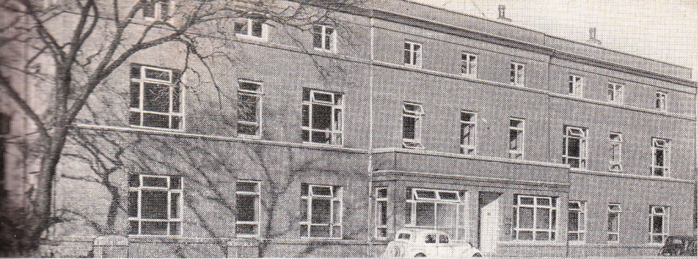
The headquarters building of Bob Martin Ltd. at Southport
